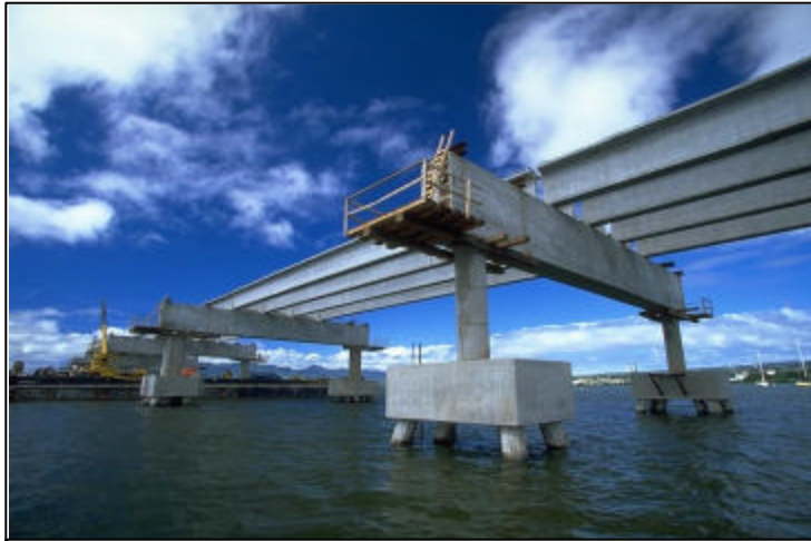
Water Line Footings in Completed Form
