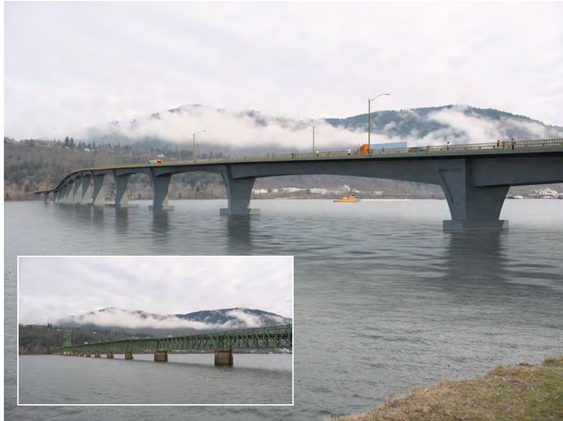
Artist rendering of the concrete segmental box girder bridge from Oregon, looking toward Washington. Inset: Original photo used to create rendering.
